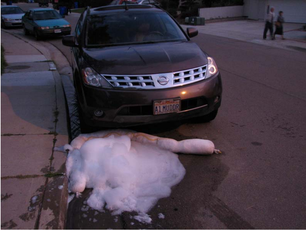
Photograph 2: Hydrocarbon absorbing boom in storm drain down hill from the crash site.
