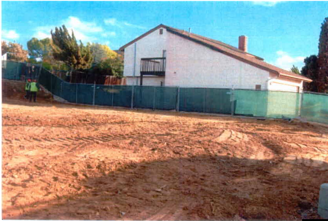
Figure 10. Site after final clean-up afternoon 14 December 2008.
