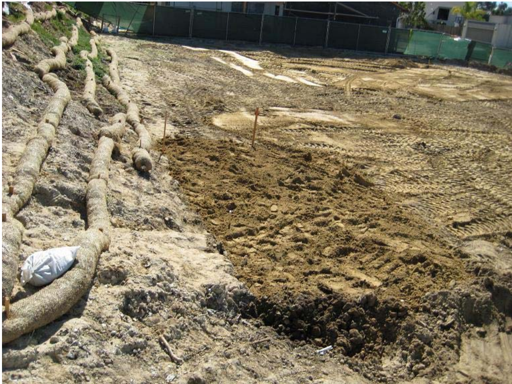
Photograph 6: Complete view of excavation area
