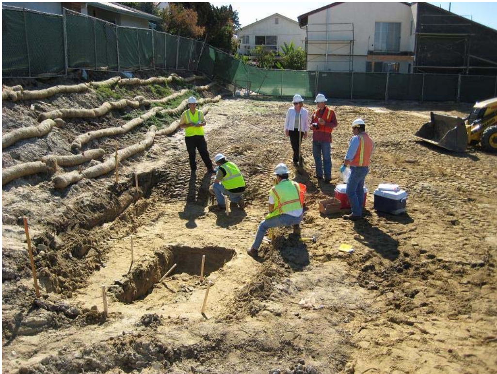
Photograph 4: View to the south of limited soil excavation.
