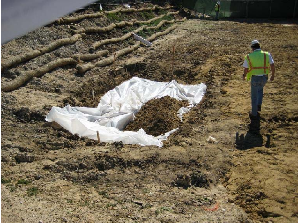
Photograph 5: Filling in excavation
